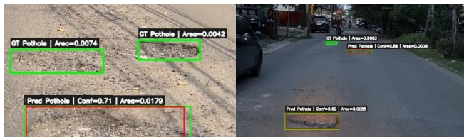
Figure 9. Representative False-Negative Cases in Pothole Detection
