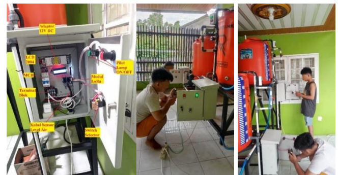
(a). The inside of one of the panels (a). Reservoir A and Main (b). Reservoir A dan B
