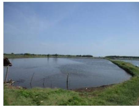
Figure 6. Condition of traditional ponds with high embankment in Donorojo District
