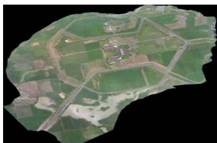
Fig.4. Aerial Photos in Kotabaru, Lampung (Suroso, I and Irmawan, E., 2018)
