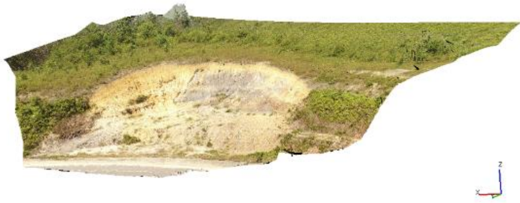
Fig. 4. Aerial view of Landslide Potential.
