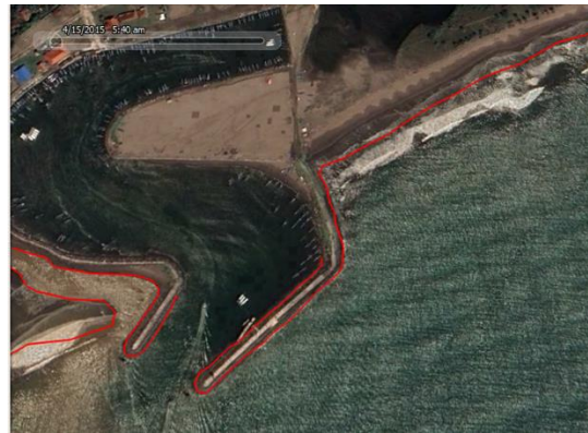
Figure 7. Coastal Coastline of the Eastern Breakwater Area of Cikidang Fishing Port
