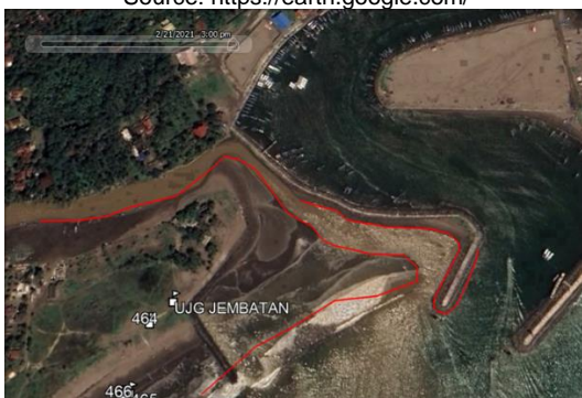
Figure 6. Coastal Shoreline of the Area Surrounding the Current Western Breakwater
