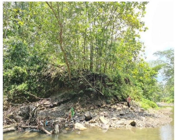
Figure 2. Landslides occurred in areas along the Karanggayam River
