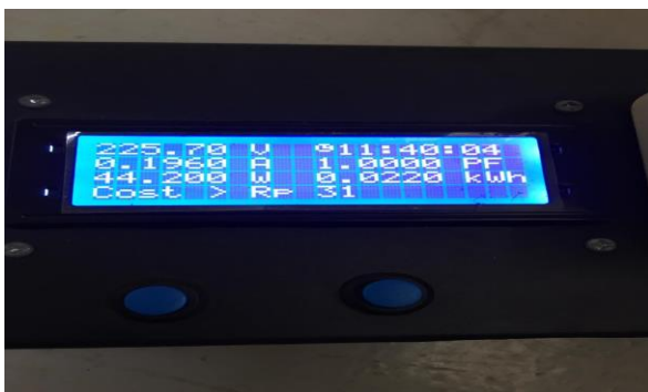
Gambar 11. Pengujian Monitoring Daya
